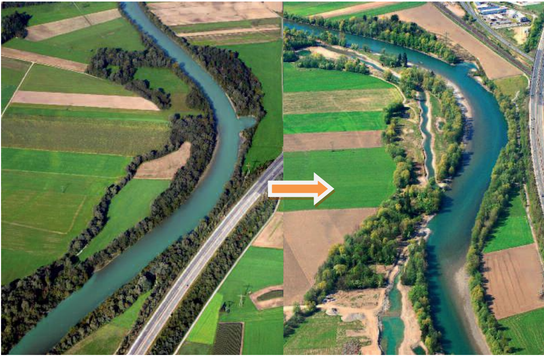
Figure 1 Before-After: The LIFE Project measure at Amlach/ St. Peter before construction in 2009 and after completion of the measure in 2011 (Carinthian state government (ed.) 2011)
