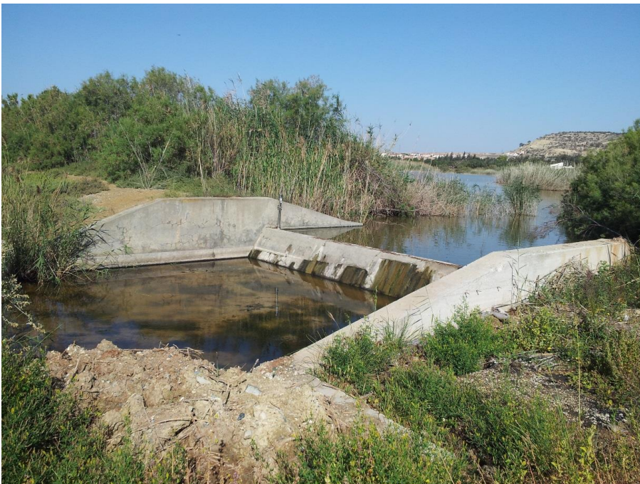
Figure 2 : The sluice was abandoned and partly destroyed, and therefore water was released in the lower parts of the wetland. In 2012, the sluice was repaired in the framework of a Life+ project and the retention capacity of the upper basin was increased. Photo: IACO Ltd (2013)
