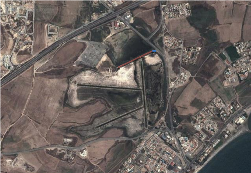
Figure 1: A small earth-fill retention dam (shown with red) and an overflow sluice (shown with blue) were constructed in 1940, in order to retain water in the upper basin of the lake and prevent its desiccation. These were constructed in order to prevent water from spreading in the lower basin, create conditions favouring mosquitos. Photo: Google earth
