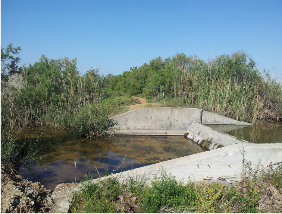
Figure 3 : The earth embankment is about 292m long and has been covered with dense vegetation. Photo:IACO Ltd (2013).
