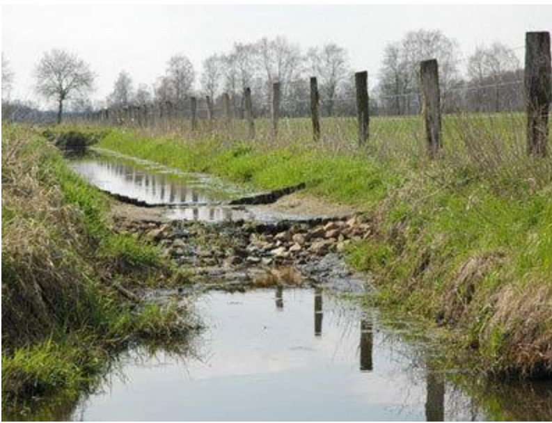
Figure 2 Overflow congestion in the project area (right from the ditch a newly constructed fence line) (Source: NLWKN)
