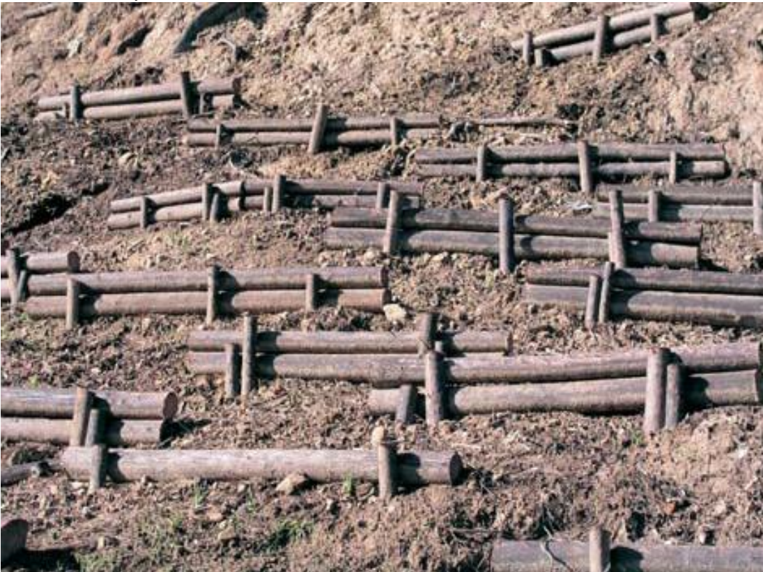
Picture 3: Detail of the timber structures (26-11-2007) (Lyrintzis Georgios, 2011)
