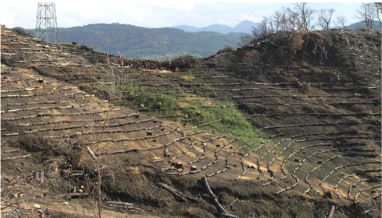
Picture 1: Kronios Hill after the implementation of the measures, Continuous Lines (Bourletsikas Athanasios, 2014)
