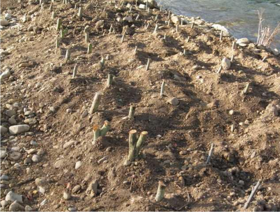
Figure 4 Works to improve longitudinal continuity: revegetation with riparian vegetation
