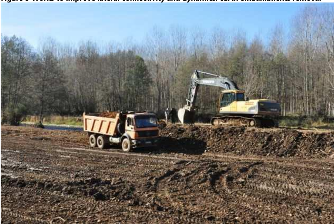
Figure 3 Works to improve lateral connectivity and dynamics: earth embankments removal
