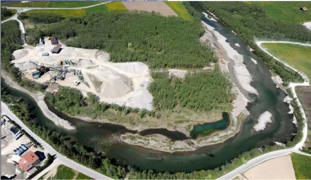
Figure 4 The riverbed after interventions (both Lot I and Lot II)
