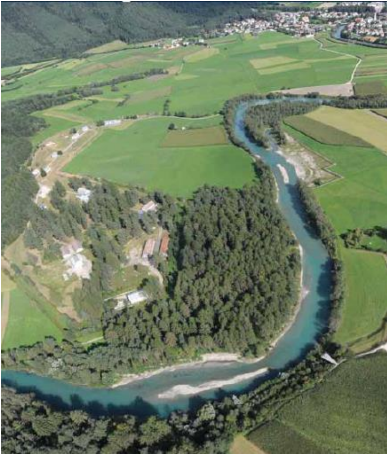
Figure 6 The riverbed after interventions
