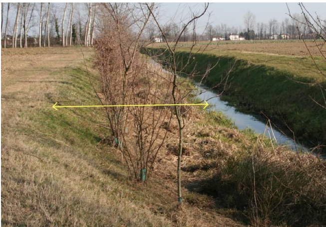
Figure 1 Buffer zone on the Piovega di Scandolara channel. The yellow arrow indicated the area where the bank was enlarged –originally, it looked like the opposite bank
