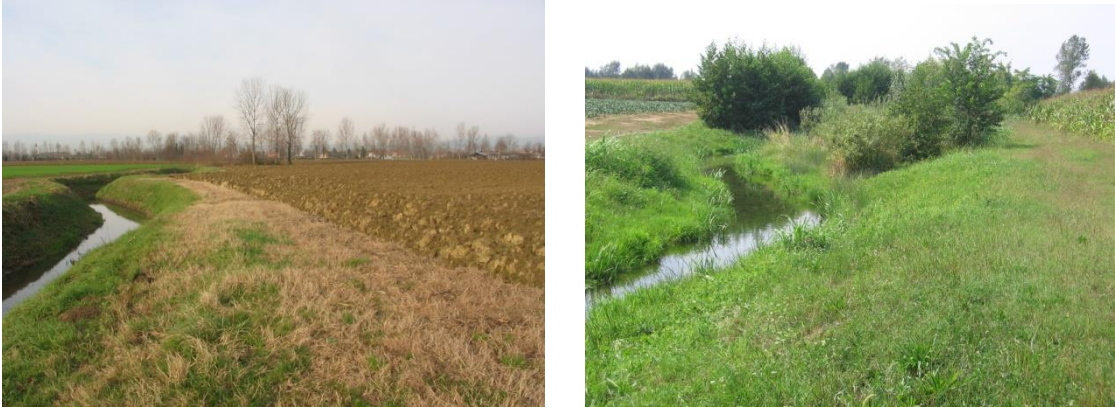
Figure 5 Scolo Desolino before and after re-meandering, river-bed widening and biodiversity improvement
