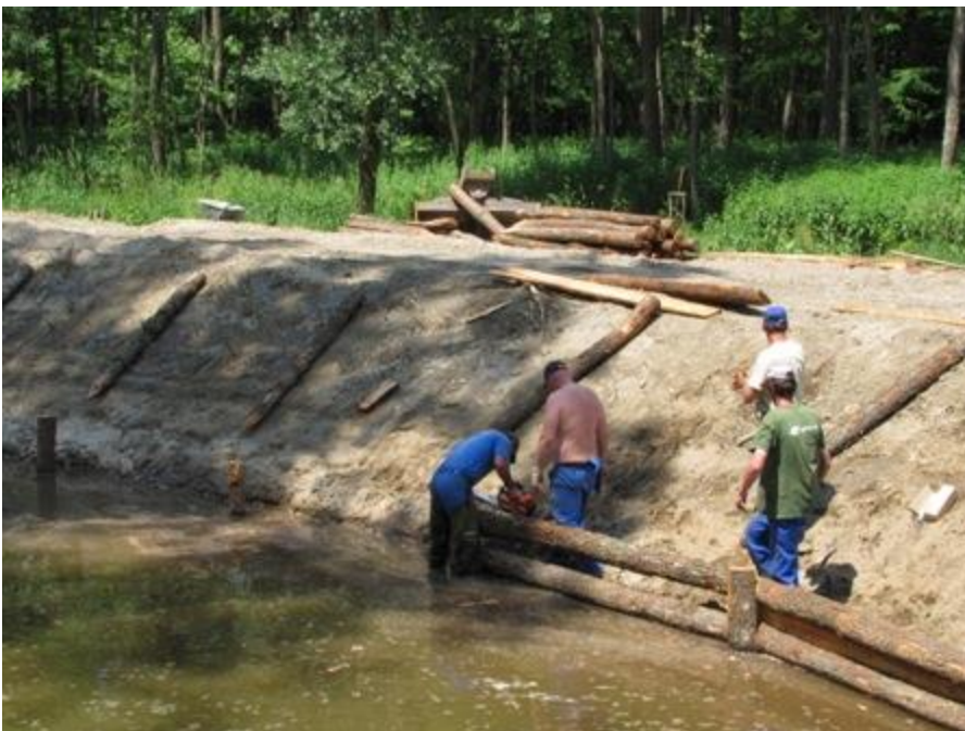
Figure 2: Working on the sidebanks (© Andrej Biro, Mura-VGP d.d.)
