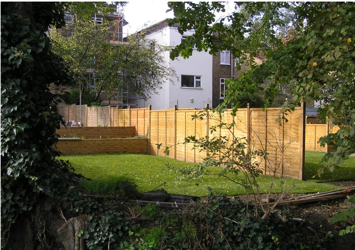
Set back flood defences in private gardens, downstream of Manor Park. Photo provided by Dave Webb, Environment Agency
