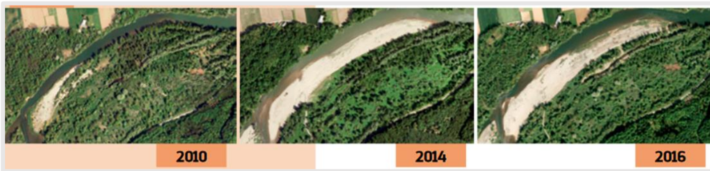
Work on the river bank and aerial photos before and after restoration (Source: LiveDrava layman's report, 2018)
