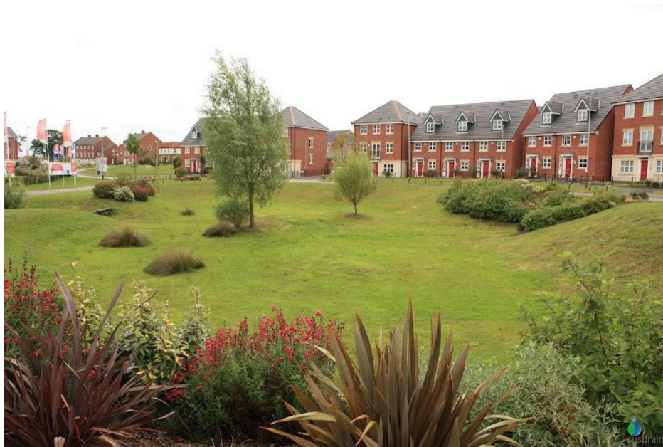
Example of a detention basin in Leicester, UK (photo courtesy of Susdrain)
