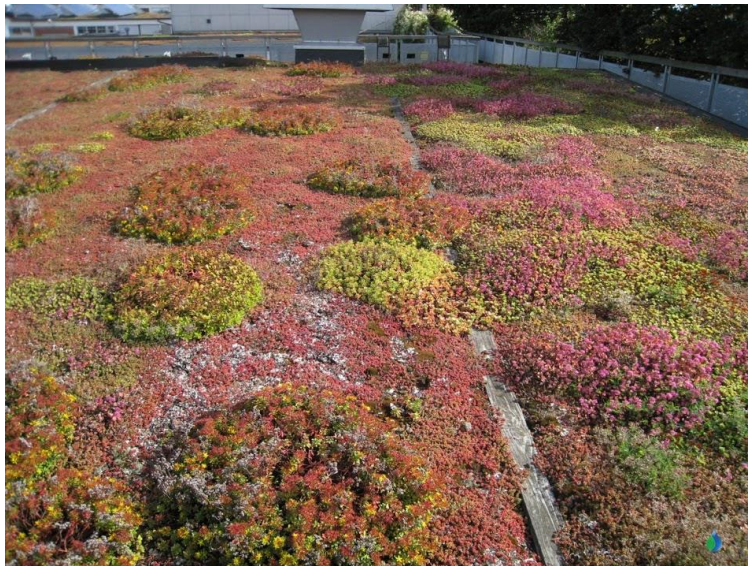
Example of extensive green roof in Augustenborg, Malmö, Sweden (photo courtesy of susdrain.org)
